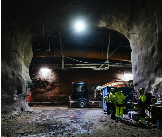
Construction is underway at the ONKALO nuclear waste repository excavated deep in the Olkiluoto bedrock in Finland. (Source: Posiva)
